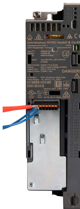
Fixing of the connections (third hand)
