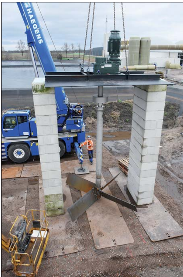
The agitators were assembled on site...
