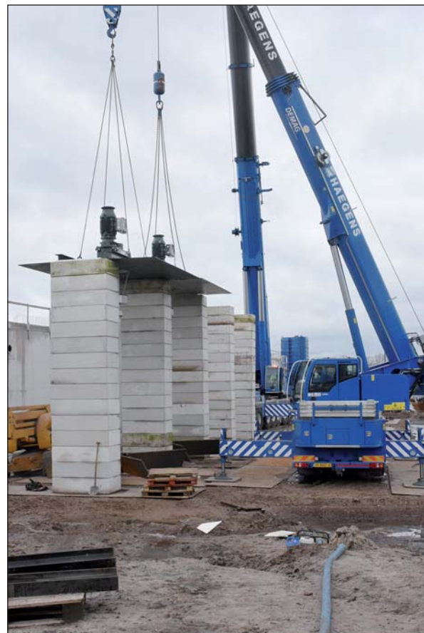
...and lifted into place with a crane.
